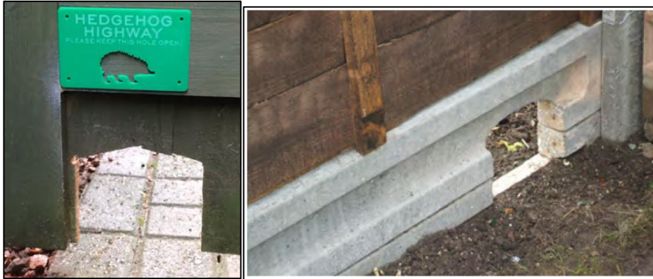
Figure 8: Examples of Hedgehog highways' that can maintain habitat connectivity for hedgehogs in residential developments
